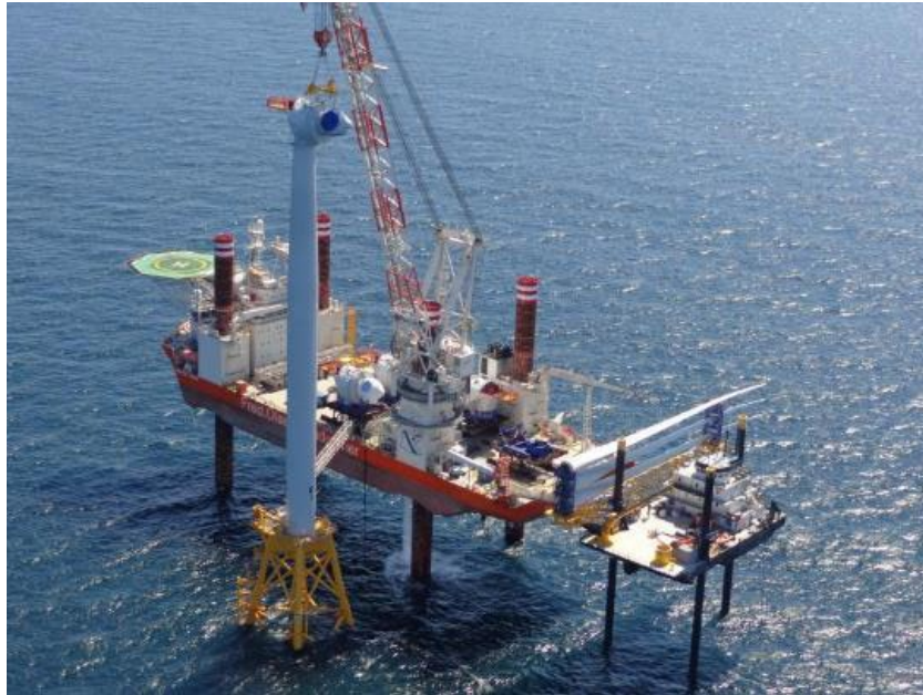
Figure 3-17. Offshore WTG Installation Vessel Source: blockisland.com
