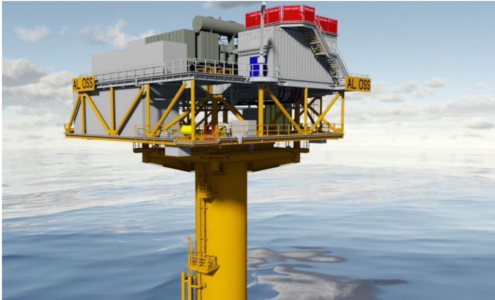
Figure 2-6. Design of Conceptual OSS atop a Monopile Foundation
