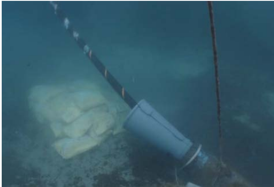
Figure 3-13. Underwater View of Near Shore Cable Pull into HDD Duct Source: Nexans.com
