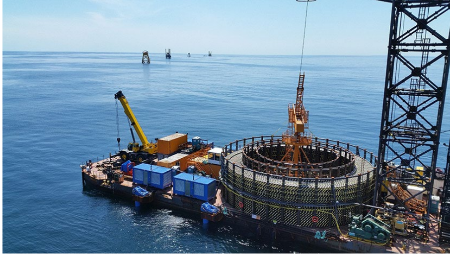
Figure 3-6. Block Island Cable Installation Source: www.oceannews.com
