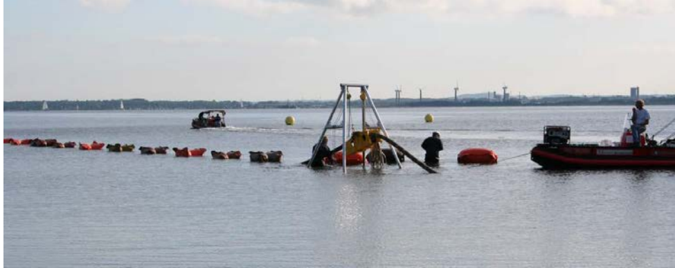
Figure 3-7. Example of Shallow Water Cable Installation
