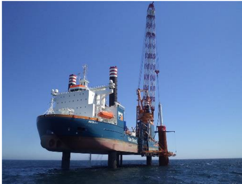
Figure 3-2. Monopile Installation Source: Globalenergyworld.com
