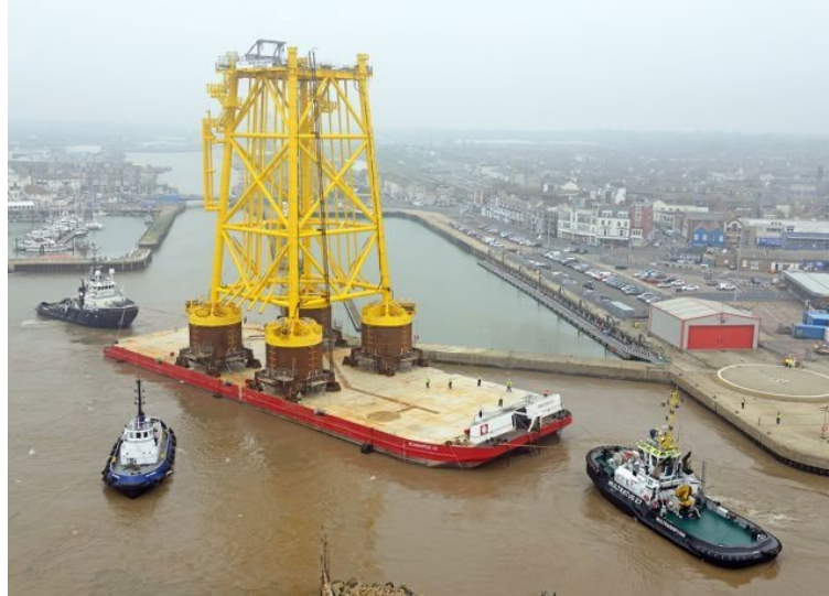
Figure 3-4. Jacket on Suction Bucket Transport Source: www.chpv.co.uk
