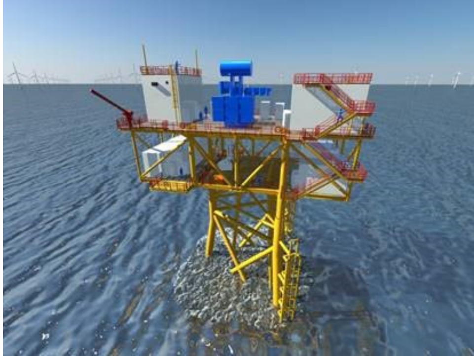
Figure 2-7. OSS on Jacket Foundation Source: HSM Offshore
